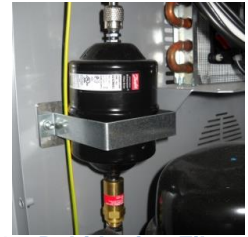
Image 51 – Dehydrating Filter
